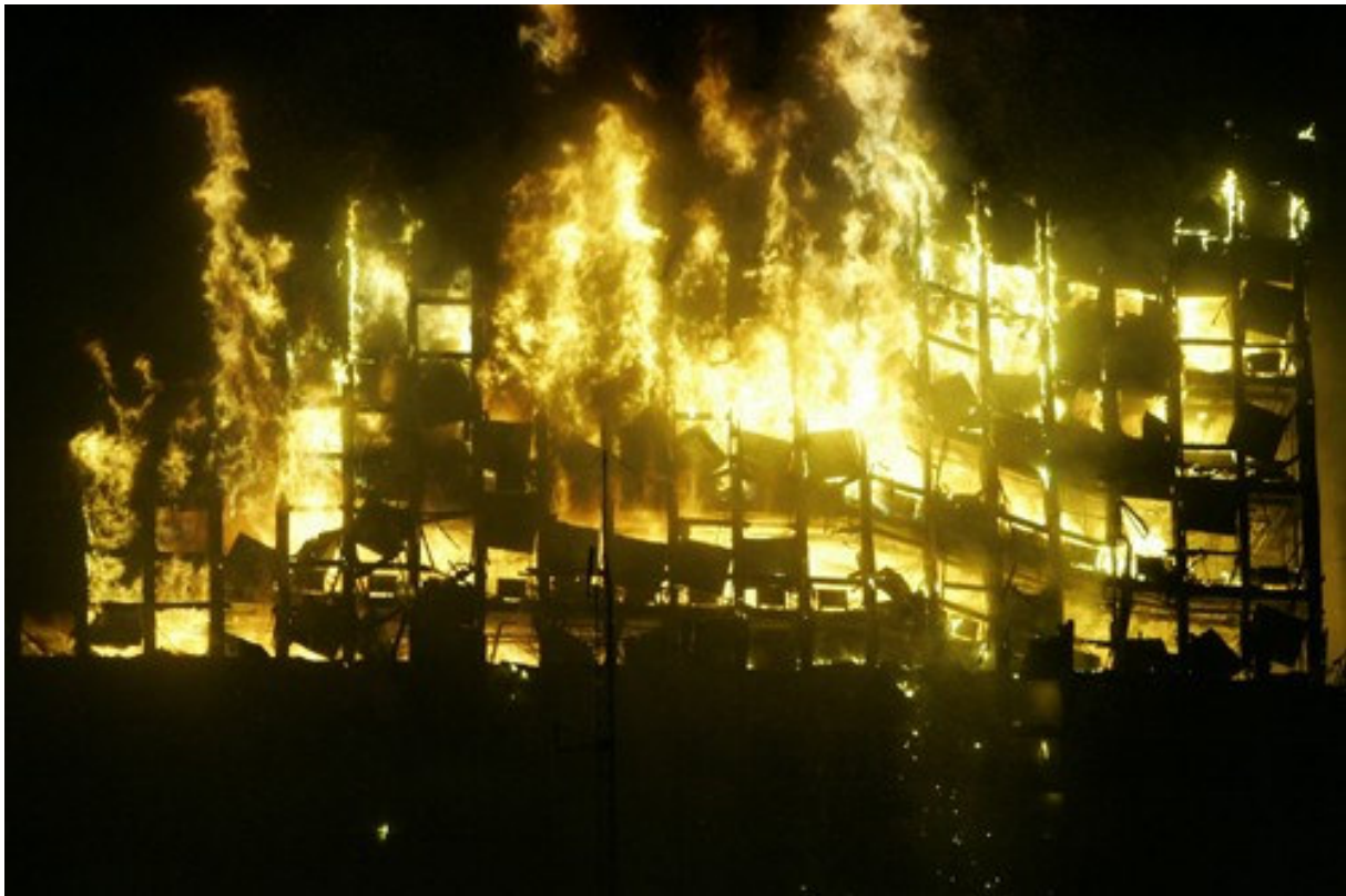
East façade as northern end collapses
